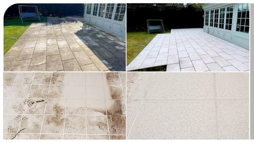
The left-hand photos show the 'before' pictures which illustrate how there can be a haze over the tiles after installation. The right-hand picture shows the tiles after cleaning, as they should be.
