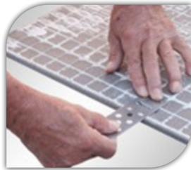
Install appropriate steel plate.
