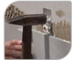
Fix steel plate to substrate using appropriate fixings.
