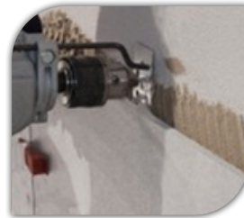
Fix steel plate to substrate using appropriate fixings.
